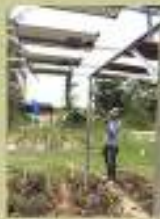
Figure 3 Solar PV system installation above the corn plot
