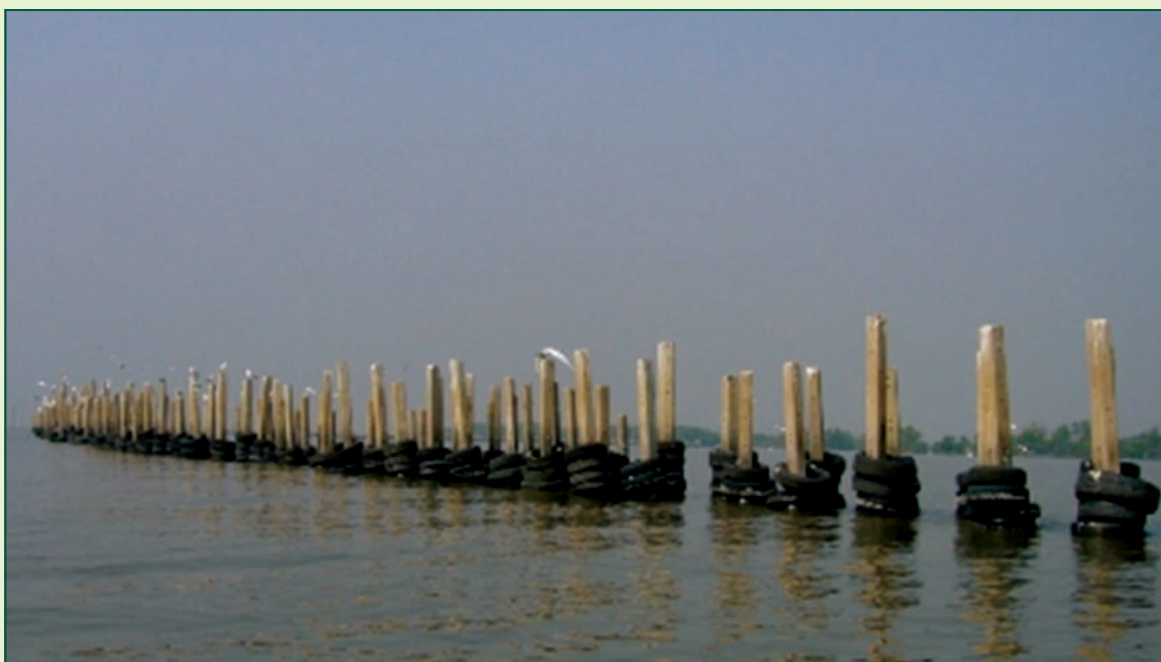
Figure 3. Bordered poles (old electric cement posts covered with old car tires) installed in the mud flat at Ban Laem Fa Pah, Samutprakarn Province decrease wave velocity and prevent coastal erosion.
