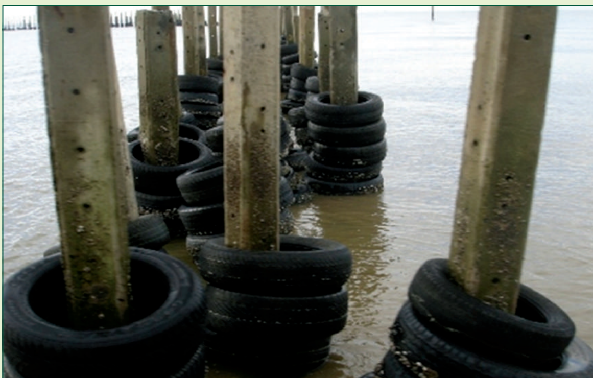
Figure 4. Three rows of old electric cement posts with seven layers of old tires can decrease wave velocity by 50 per cent and prevent coastal erosion.
